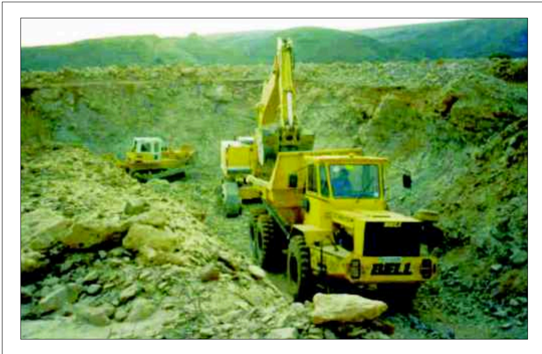
Figure 13 – Pit excavation – Middelwater Project
